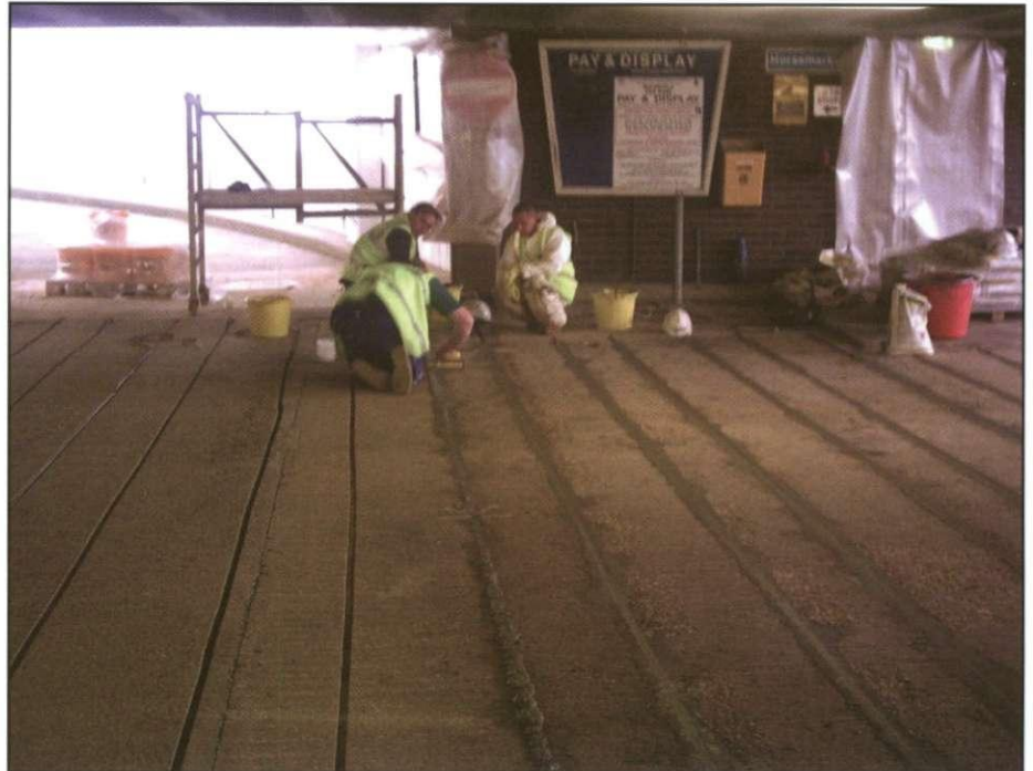
Figure A4 Installation of anodes in deck.
