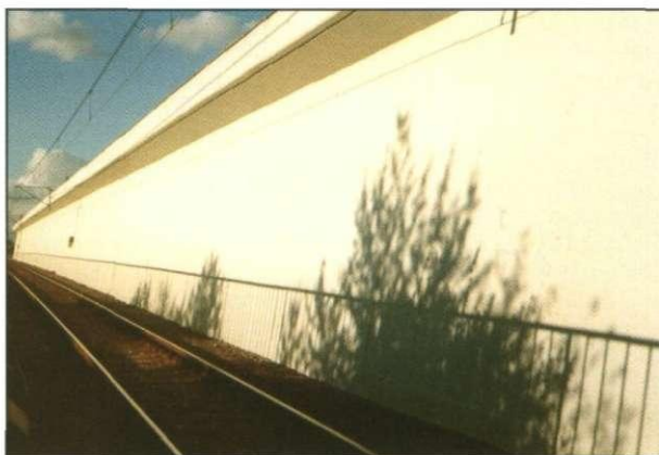
Figure 4 Surface coating applied to repaired structure.
