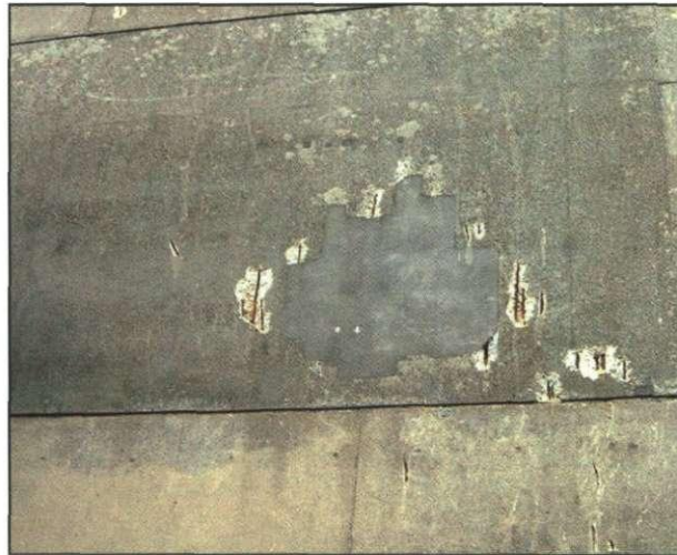
Figure A9 Incipient anode formation.
