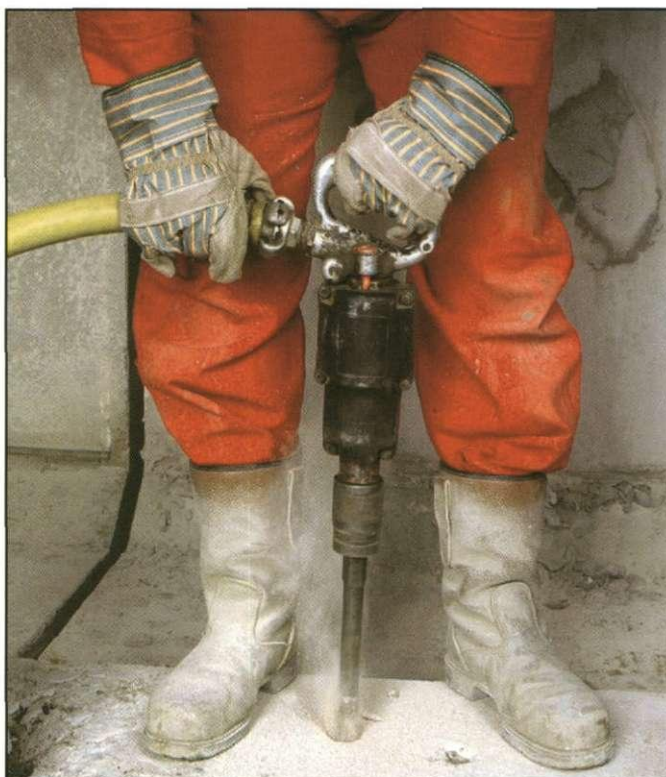
Figure 9 Hole drilling using rotary percussive air flush drill bit.
